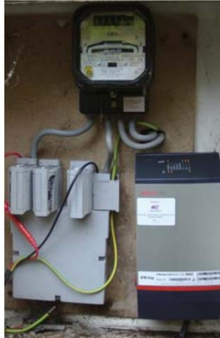
A repeater installed in a customer's meter box at a Power Line Telecommunication (PLT) trial installation. For this particular system the repeater was required to translate data signals in the 1.9 to 11.3MHz band from the street cables up to 18.7 to 25.1MHz for in-house distribution. Note that the repeater input and output share the same wires and there is no filtering to separate the street signals from those indoors. For economic reasons this feature is common to both in-house and access PLT.
